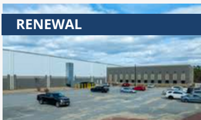
DEVENS, MA 36 Saratoga Boulevard 162,000 SF to New England Sheets
