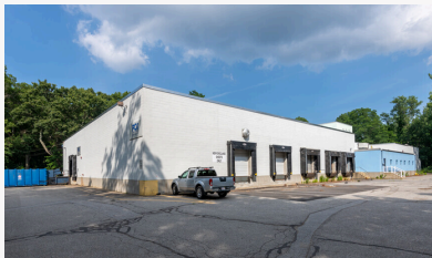
LEASE 33 Glen Avenue, Chelmsford 36,000 SF InfraServices Group
